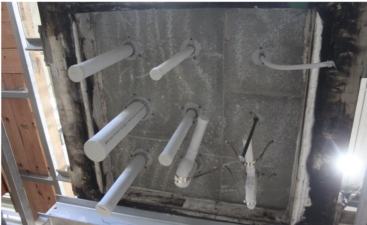
Figure 30 – Exposed face prior to test commencement
